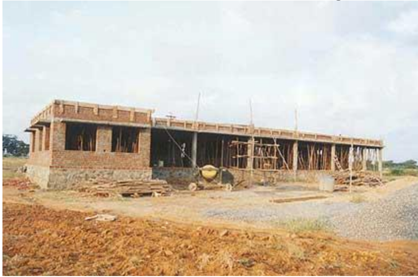
Front view of Non-Formal Education Building:
