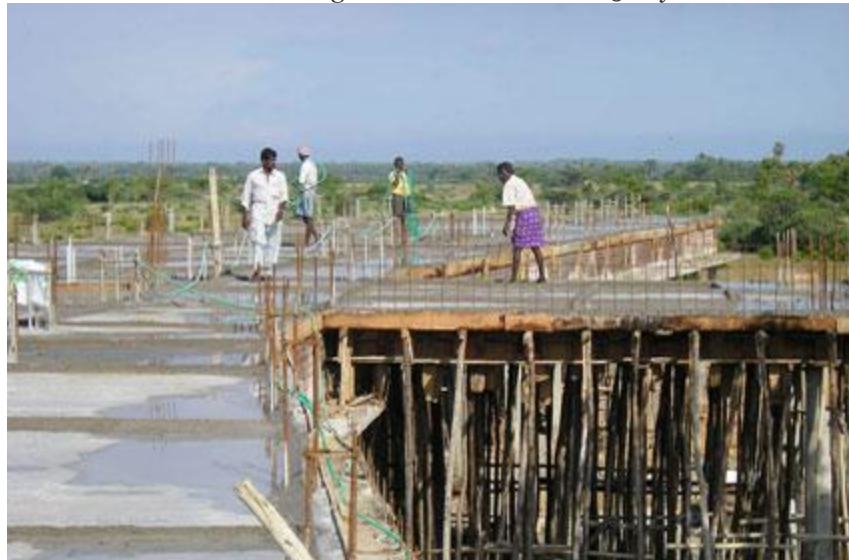
Concrete being cured with water for 25 days:
